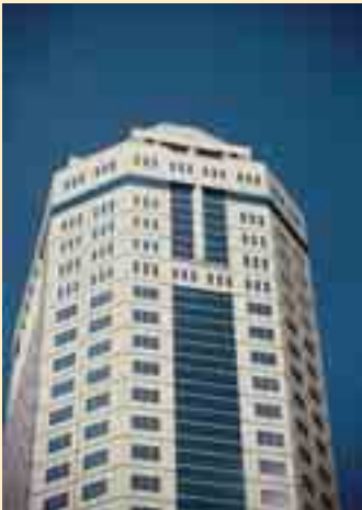
State Office Tower II, in Columbus, Ohio, has 3 cm of granite on 5- and 7-inch-thick precast concrete backup. (Architects: Bohm-NBBJ)
