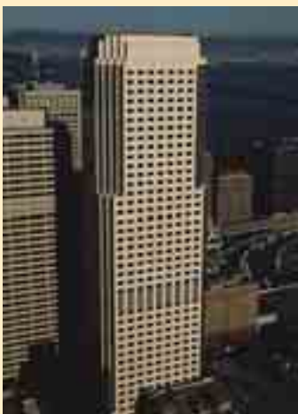
Five Fremont Center in San Francisco is clad with 1 1/4- and 2-inch-thick travertine-faced precast concrete panels. (Architect: Skidmore, Owings & Merrill)
