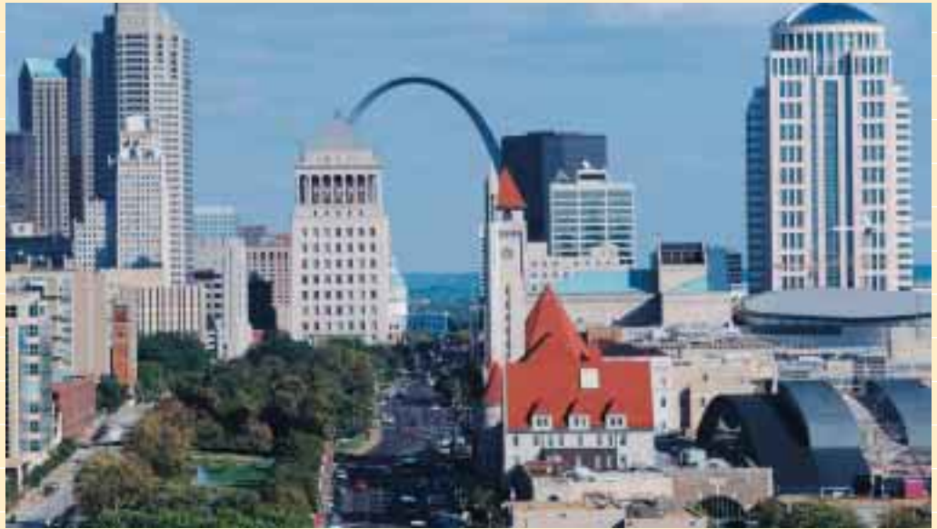
The multi-color precast exterior of the 29-story Thomas F. Eagleton United States Courthouse, St. Louis, Mo., stands out as one of the most unique skyscraper dotting the skyline.
