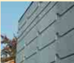
This close-up shot of precast panels at the Ft. Eustis Aquatic Center shows the building's strong horizontal reveals in wave shapes adjacent to vertical panel joints
