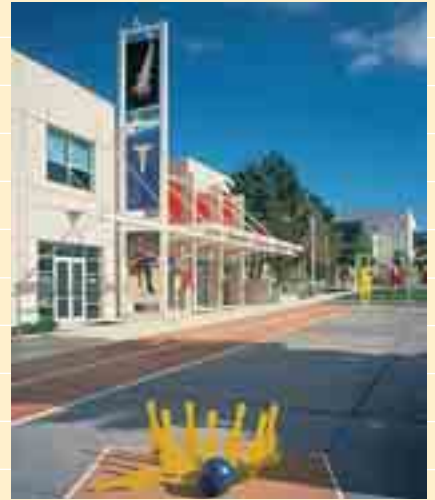
The Sports Medicine & Technology building and the new Sports Exhibition Center entrance feature horizontal and vertical reveals designed to work in conjunction with major building openings and the vertical and horizontal precast fins that create an entrance canopy.
