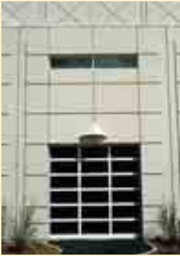
This detail of the U.S. Olympic Gymnasium shows the operable garage door leading into the weight-training area. The space was designed with a pattern of vertical and horizontal reveals on the structural bay and the window articulation. The diagonal reveals of the building's main body can be seen beyond.
