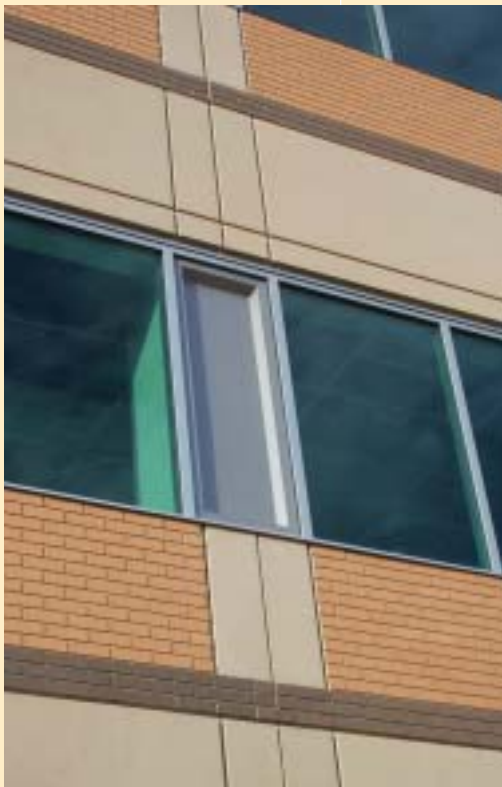
Close-up of orphaned light-colored, thin-brick units at accent field to vertical exposed precast column cover transition. Photo: courtesy of Gensler.
