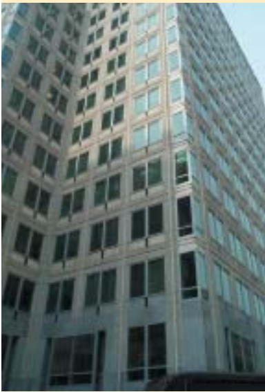
Example of black granite stone clad precast inset accents on architectural precast and glass and metal clad high rise office building.
