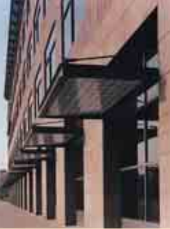
Orchestra Place Office Building in Detroit used precast panels to achieve a traditional, solid look.
