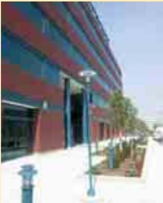
Oakland Commons Office Building in Southfield, Mich. features CFPCP to alternate with bands of glass to create a distinctive, contemporary look on an economical budget.
