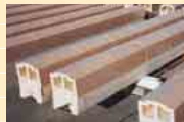
Fig. 7: One-inch-thick brick cladding on 5-inch-thick concrete panels was used on the first three floors of the Sacramento County System and Data Processing Building in Sacramento Calif. Terra-cotta medallions were placed on spandrels and column covers. Architect: Ehrlich-Rominger
