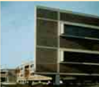
Fig. 5: Spandrels and wall panels on the Sylvan Corporate Center in Englewood Cliffs, N.J., have integrally cast 8-inch-square brick-colored tiles with pigmented mortar. Architect: Herbert Beckhard Frank Richlan & Associates
