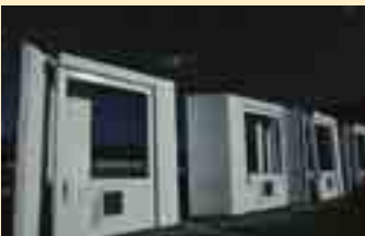
Fig. 4: These panels have 6-inch-square glazed white ceramic tiles and some additional 10-inch-square accenting blue tiles.
