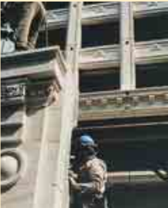
Fig. 6: Built in 1906, the architectural landmark 88 Kearney St. in San Francisco had its terra cotta removed and reassembled on precast panels for an all-new structure of taller height. Architect: Skidmore Owings & Merrill
