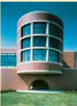
Fig. 1: Radial brick was cast into radiused precast concrete panels for the S.C. Johnson Worldwide Professional Headquarters in Mt. Pleasant, Wis., to create the smooth flow around corners. Architects: Zimmerman Design Group and Hellmuth, Obata & Kassabaum Inc.
