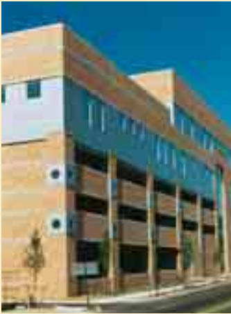
Fig. 11: The perimeter columns and wall components of the St. Peter's Ambulatory Surgery and Parking Structure in New Brunswick, N.J., were cast with dovetail slots to facilitate quick installation of full brick in the precaster's yard. Architect: Desman Associates Photo: @Robert Mueller Architectural Photography
