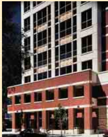
Fig. 7: One-inch-thick brick cladding on 5-inch-thick concrete panels was used on the first three floors of the Sacramento County System and Data Processing Building in Sacramento Calif. Terra-cotta medallions were placed on spandrels and column covers. Architect: Ehrlich-Rominger
