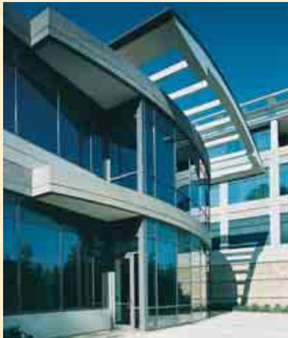
Fig. 4: This flat wall plane on the 55 Farmington building in Hartford, Conn., changes direction without corner articulation by using a shallow angle return for single casting and placing the joints at the back angles where they are de-emphasized. The shallow corner angle allows a solid cast edge.
