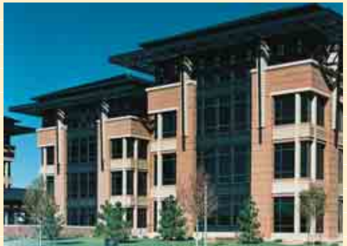
Fig. 3: Two-stage cast covers with deep returns were used for the solid-block treatments of piers at the Merrill Lynch Campus in Denver. The two-stage precasting allows a unique cast-in surface texture to be carried around the corners of the blocks to a much deeper dimension. Minimal corner dry joints without quirks complete the appearance of a solid unit.
