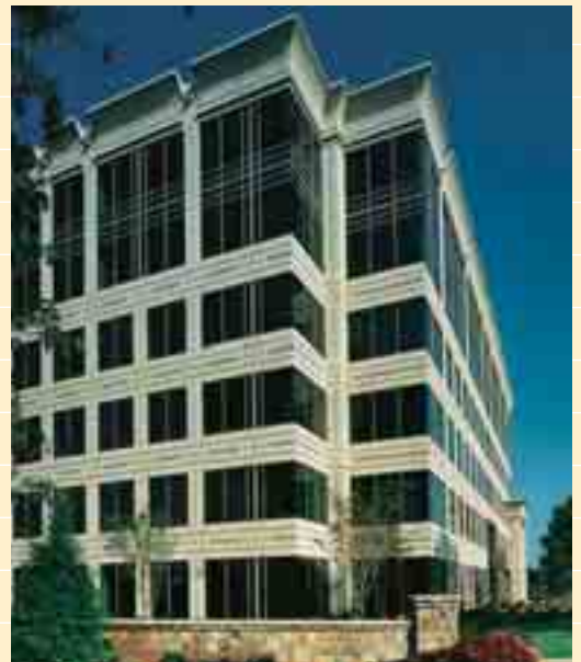
Fig. 7: The minimal quirk miter corner in the spandrel panels at the Metropolitan Life Building in Atlanta provides an uninterrupted planer return of the profiled wall-panel surface without corner articulation. A two-stage casting at the cornice provides a similar planer wrap around the top. These sharp corners at the top emphasize the building corner's larger-scale articulation. Details closer to pedestrians use the quirk corner for more finished detail.
