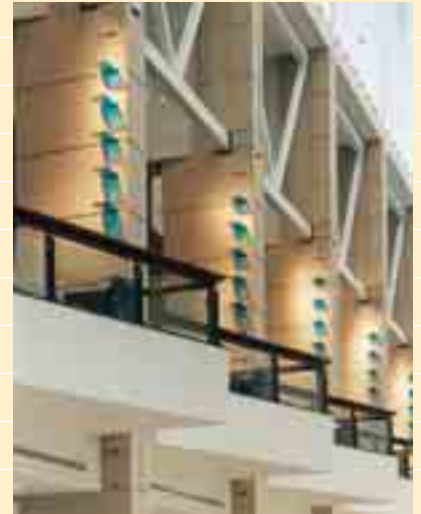
Fig. 5: The returns on these column enclosures at the McCormick Place Expansion project in Chicago aren't intended to imply a material thickness of panels or blocks but to provide a planar wrap of the surfaces forming the corner. The joint is located at the pier's center to provide a linear continuation of the element above the pier.
