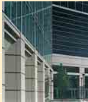
Fig. 2: On Chicago's McCormick Place Expansion project, one-piece channel-shaped covers with relatively shallow returns were used to imply a thickness somewhat more than the actual panel thickness. In this case, well-executed "sharp" corners in the casting add to the solid appearance.
