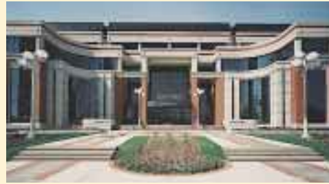
...Form a concave building corner; Molds F & H.
