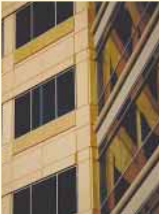
The combination of different colors and textures of precast structural spandrel panels, including radius panels, creates a highly articulated but very cost-effective façade at the 370 Interlocken Blvd. project.
