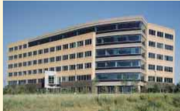
The use of curved precast panels allowed the designers to "break out of the box" at the 370 Interlocken Boulevard project in Broomfield, Colorado. Photo: Ed Lacasse
