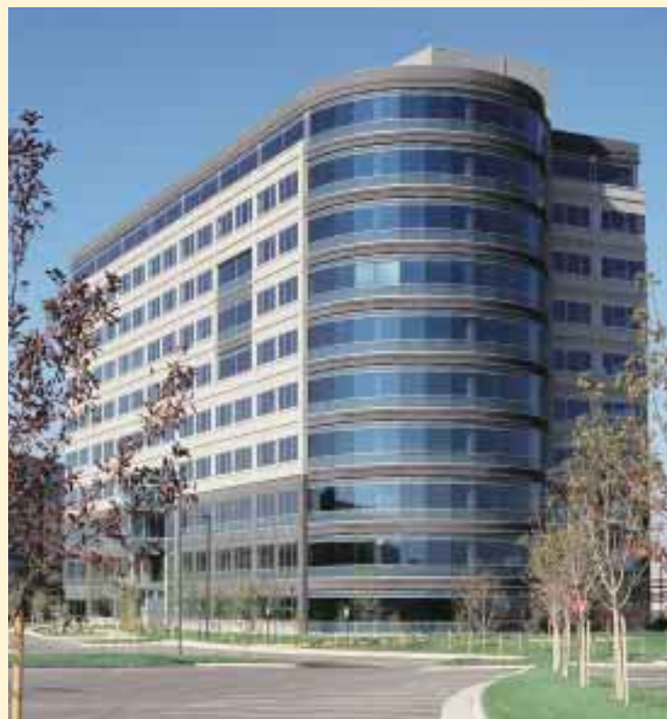
The combination of radiused structural precast panels and storefront glazing allowed designers to express a curved "glass" volume without the additional cost of the curtain wall at the 380 Interlocken Crescent project in Broomfield, Colo. Photo: Blake Mourer, Gensler
