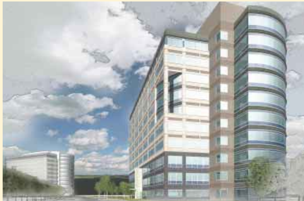
At 390 Interlocken Crescent, curved precast panels accentuated the building corners, and similar curved panels were introduced to the building's main façade.
