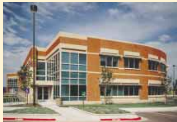
At the Jefferson County District Attorney's Office Building, masonry units cast into the precast panels provided a combination of brick and precast detailing. Photo Credit: Jun Xia, Gensler
