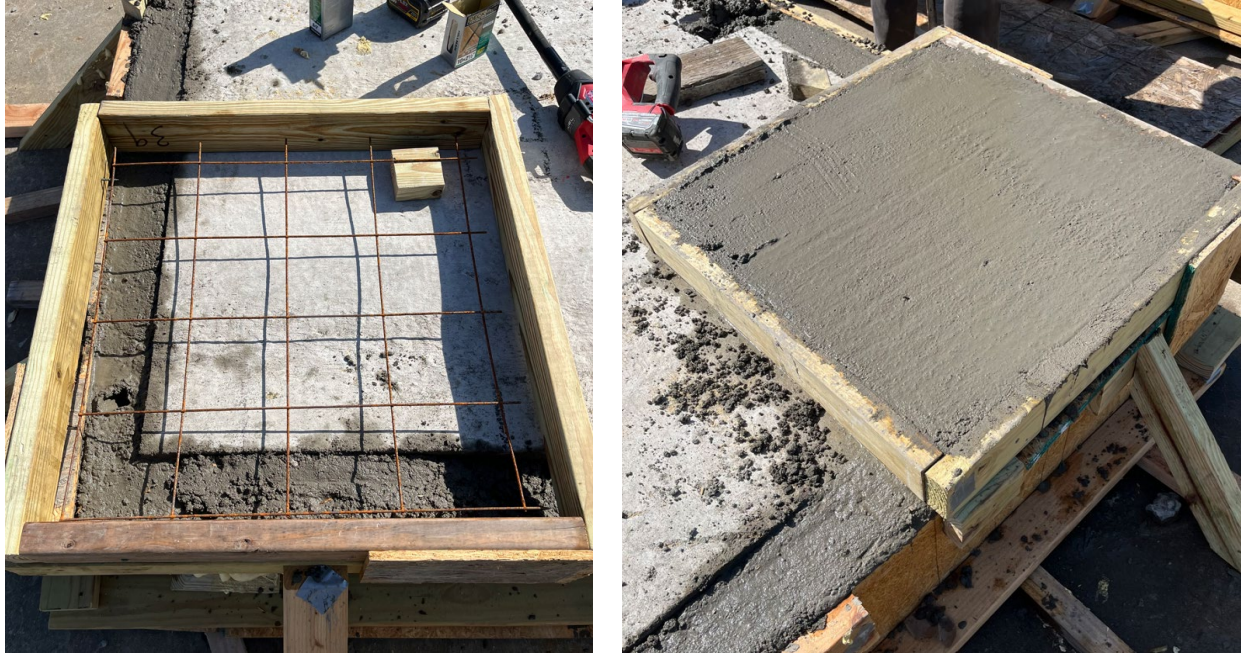
Figure 5 – Photos of topping slab placement
