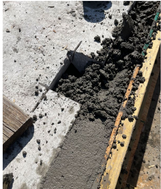
Figure 4 – Photos of edge pour construction and concrete placement
